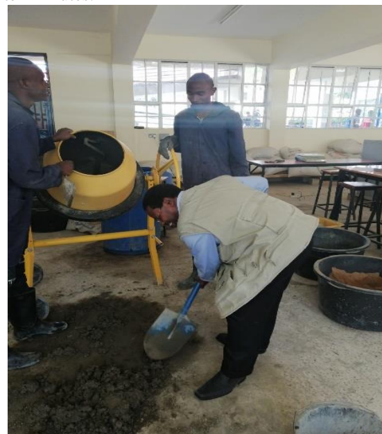
Fig 3: Hand mixing of concrete.
