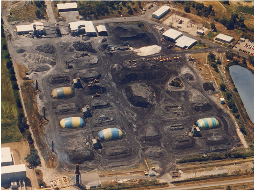
FIGURE 19.8. Exolon-ESK plant in Hennepin (Illinois). This plant is one of the newest SiC facilities in the world, producing 45,000 t of both high-quality metallurgical and crystalline SiC annually. It is North America's only manufacturer of SiC. The plant features 16 furnaces operating off of four transformers.
