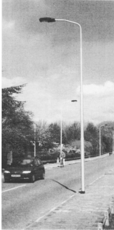
Fig. 9.4 Lamp post in Pijnacker (the Netherlands).
