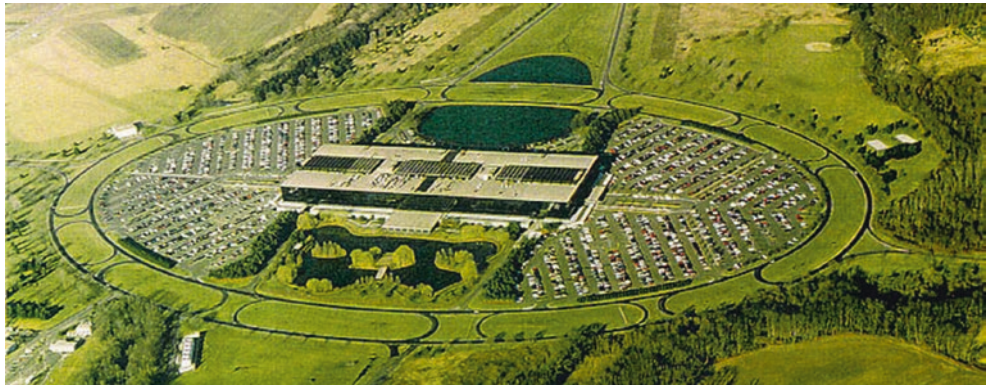
Fig. 4.1 Bell Labs R&D facility in Holmdel, NJ
