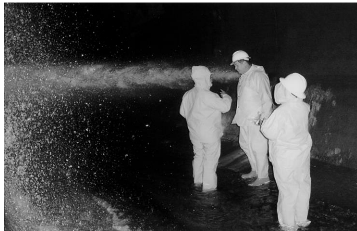
Fig.19: Encounter with underground water problem
